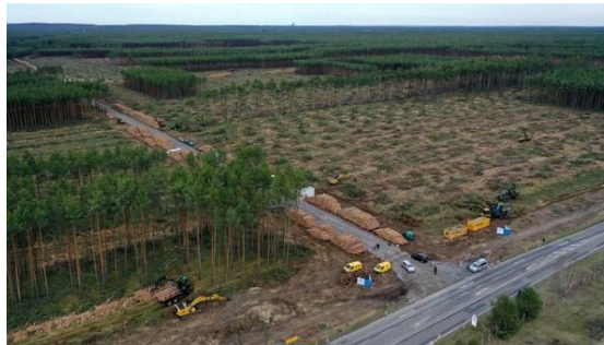
Picture 1: Deforestation to build a factory
